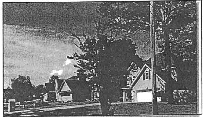
Single family residential, Newtown Church Rd.
